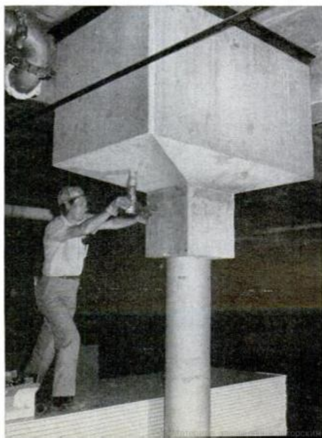
BLOCK ABOVE WORKMAN is a giant "flowerpot" for tree on surface. Valve controls the watering system
